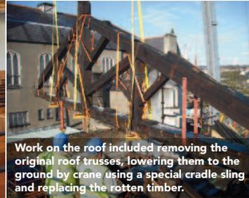
Work on the roof included removing the original roof trusses, lowering them to the ground by crane using a special cradle sling and replacing the rotten timber.
